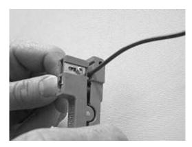
Figure 7 – Ring cut the buffer tube.
