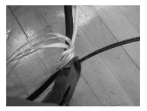
Figure 5 – Cut and remove the two sections of cable jacket.
