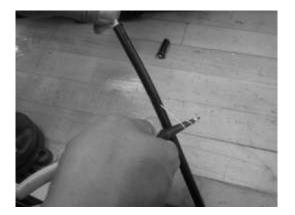
Figure 3 – Pull the rip cord through the armor and outer jacket.
